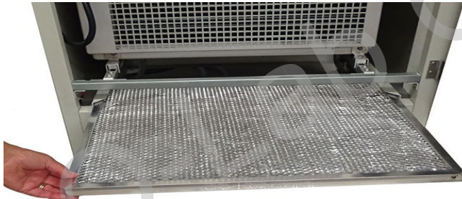
Chiller Air Filter
